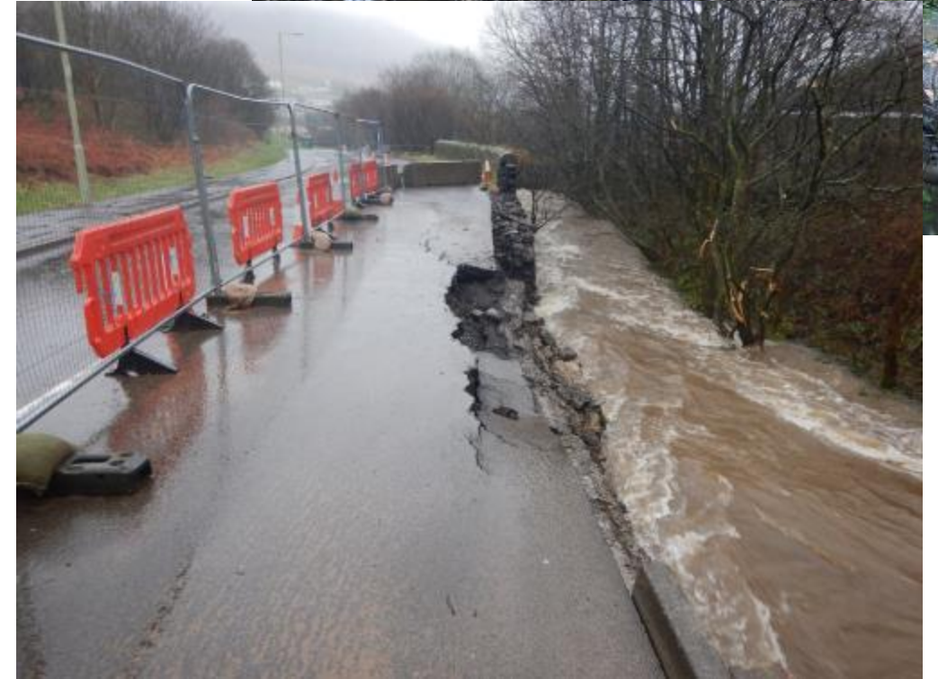
Blaen y Cwm Road Ynysangharad Park Footbridge
